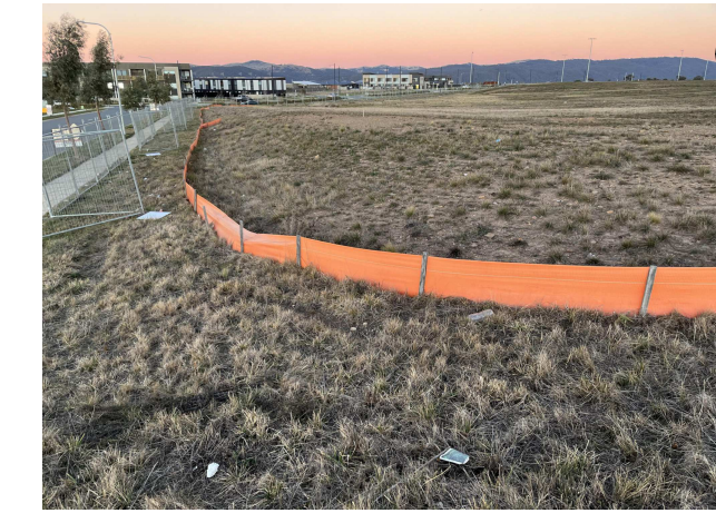
1 CORNER OF OBSERVER STREET AND GLENROCK DRIVE
